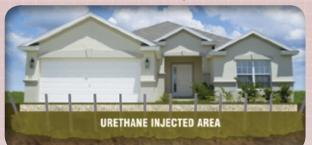
Chemical Grout Injection is a process of injecting a near waterviscosity liquid under low pressure, into cohesionless soil to create a solid stonelike mass.
