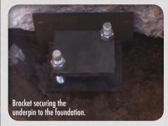
All of the foundation brackets that we install are fully adjustable. Any vertical adjustment later required can be easily accomplished with no adverse impact on the property.
